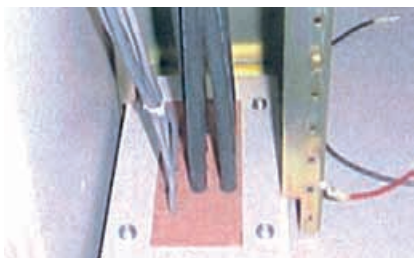
• Corrosion Protected lightweight transit is inserted into a turbine housing.
